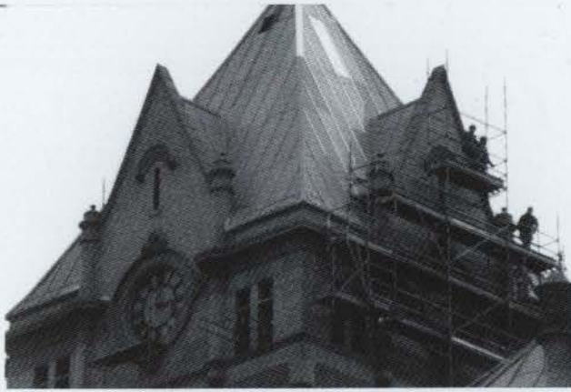
Workers renovating the clock tower, 1996
