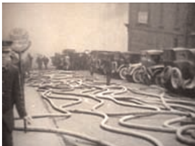
Hoses are scattered about as Detroit firefighters attempt to battle a building blaze at Wayne and Woodbridge Streets.
