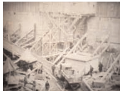
Building the foundation of the Book-Cadillac Hotel.
